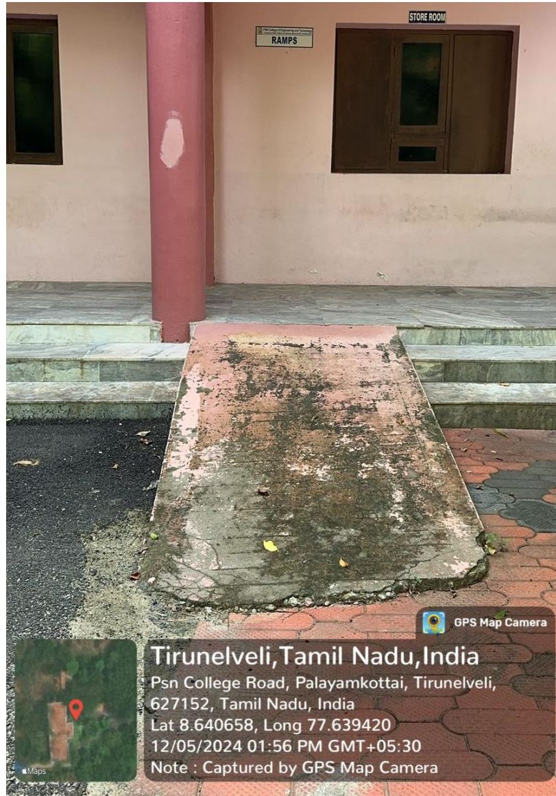
Ramps at Admin Block
