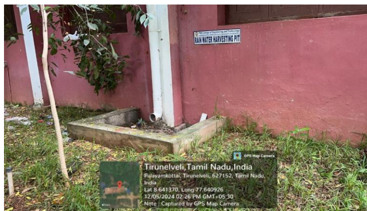
Rain water harvesting Pit in the First Year Block
