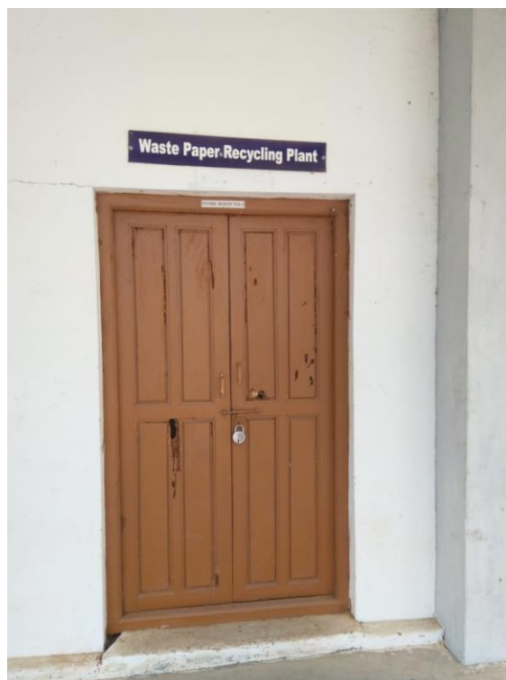
Waste recycling Plant
