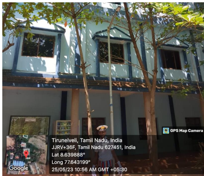
A View of Sample Light opposite to Main Building
