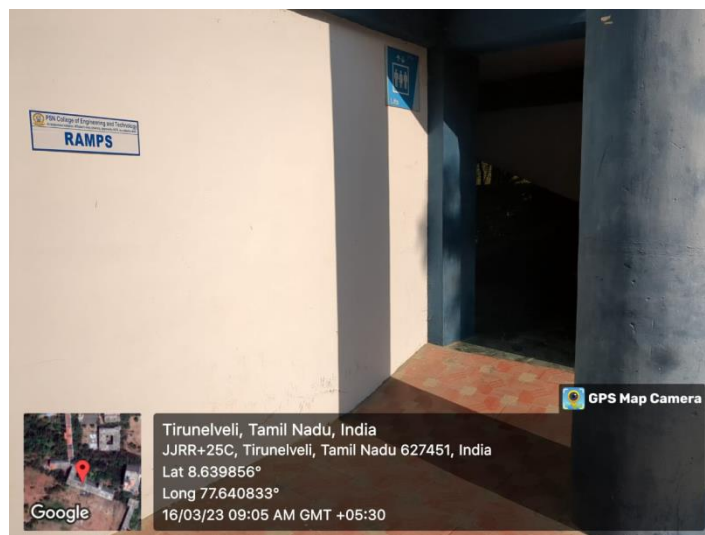
Ramp in the Knowledge Resource Center (Library) Block Ground Floor
