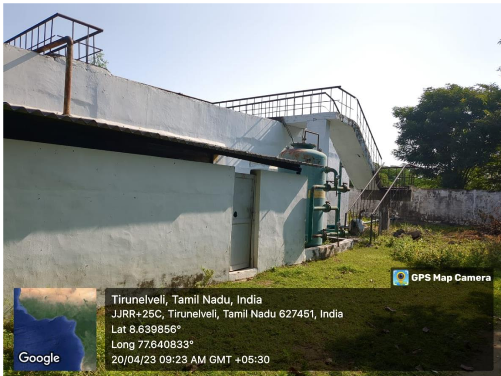
A View of Sewage Treatment Plant (STP)
